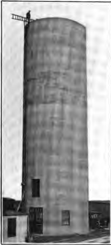
WATER TANK At Chicago Junction, Ohio, built by Steel Concrete Construction Co. for the B. & O. Railroad.
